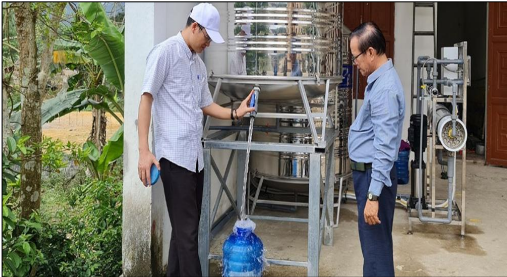
Staff testing a newly installed water system
